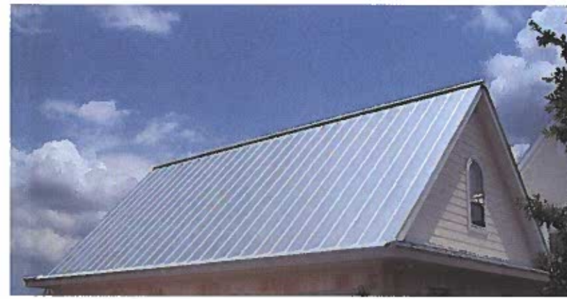
STANDING SEAM METAL ROOF
